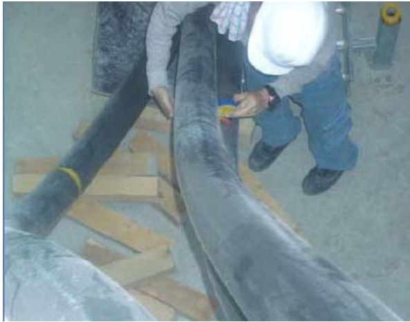
Exposure of Power cable conductor
