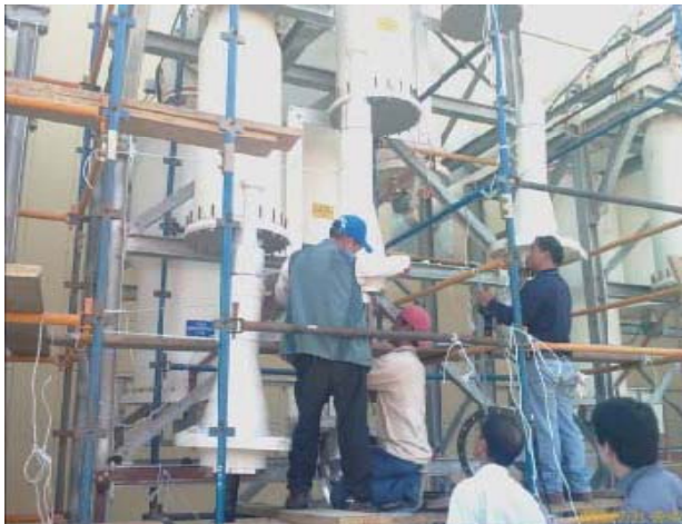
Waterproofing and application of Epoxy putty
