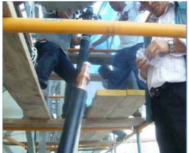
Waterproofing and application of Epoxy putty
