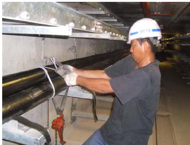
Arrangement of Power cable in the UPN Support after laying
