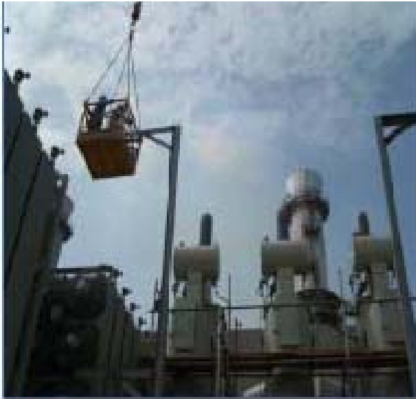
Connection set up in the Test Bushing for Transformer
