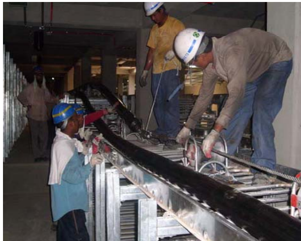
Arrangement of Power cable in the UPN Support after laying
