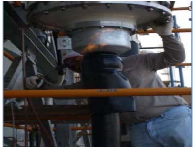
Waterproofing and application of Epoxy putty
