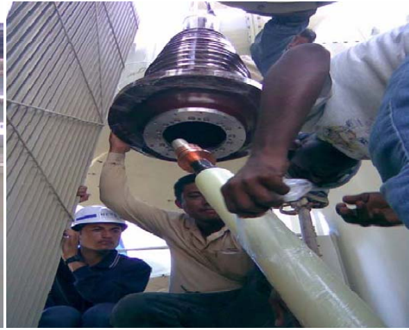
Assembled Transformer SE ready for insertion
