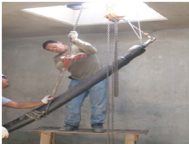
Arrangement of Power cable in the UPN Support after laying
