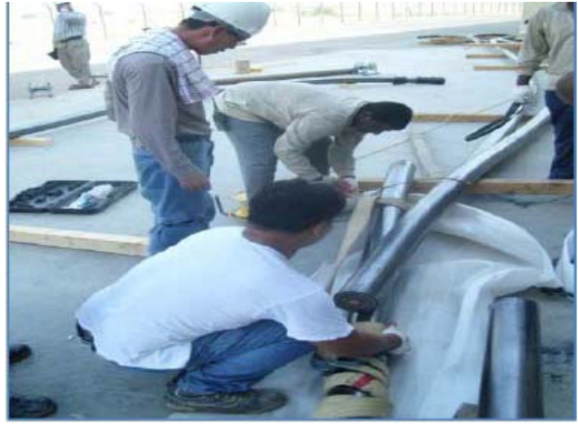
Exposure of Power cable conductor
