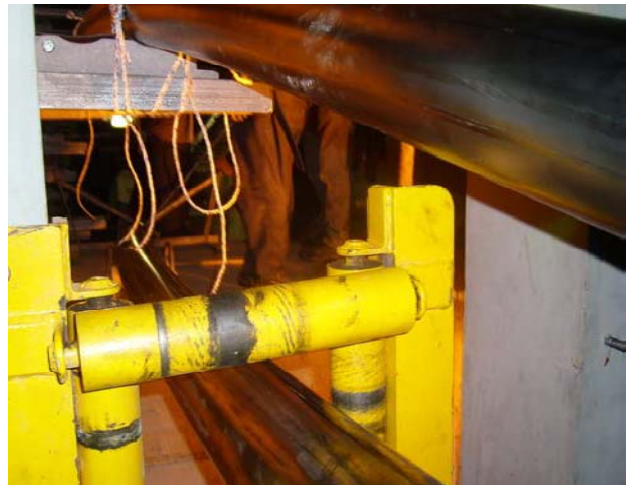
Arrangement of Power cable in the UPN Support after laying
