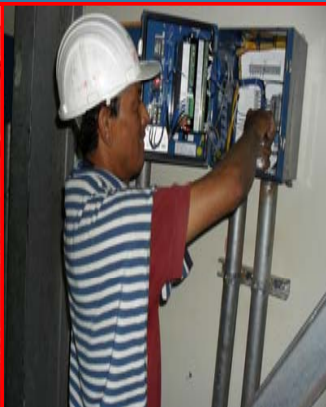
• Control Cables Termination
