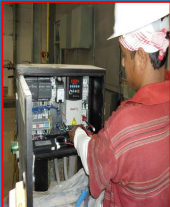
• Control Cables Termination
