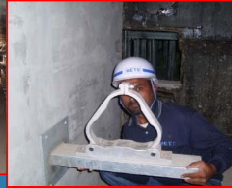
• Tripoil Cable Cleats Installation
