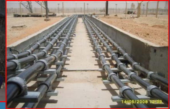
• Cable Cleats Installation
