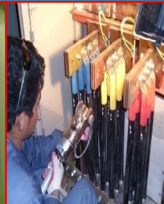
• Low Voltage Cable Termination
