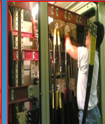
• Low Voltage Cable Termination
