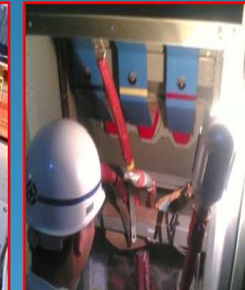
• Medium Voltage Cable Termination
